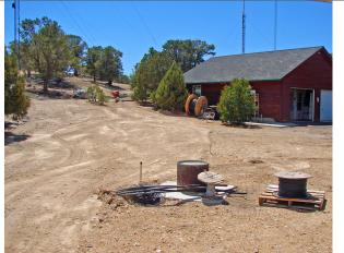
After more than a year of open trenches, the feedlines are finally buried. This is the base for the 80M Monopole (20" steel pipe in 3 yards of concrete)
