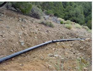
Where the ground is very rocky, the cable was laid in PVC Pipe
