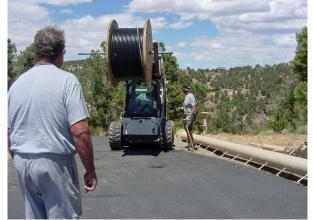
First, we had to replace old coax new 7/8" and 1/2" Heliax. W6NF and K6NV were the "pullers" for nearly 3,000' of coax and another 2,000' of replacement control cables.
