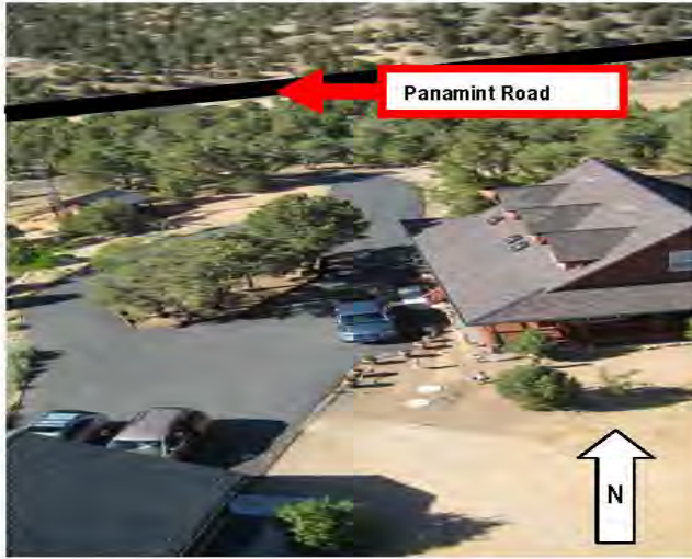
Figure 7: The paved driveway facilitates continuous circular traffic flow. Provided that the travel way is maintained free of vehicles and other obstructions, there appears to be adequate travel and staging space for emergency vehicles and other equipment.
